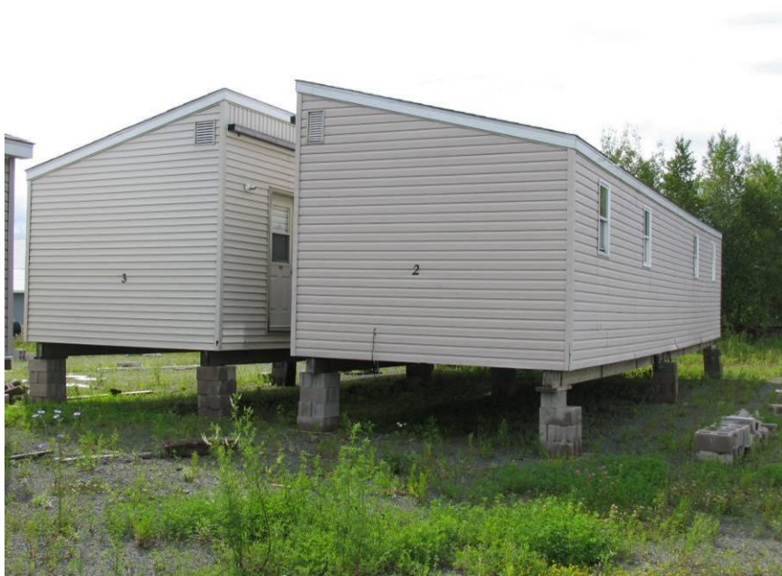
Parcel 3.16G 12' x 40' Pre-Fab Crew Quarters
