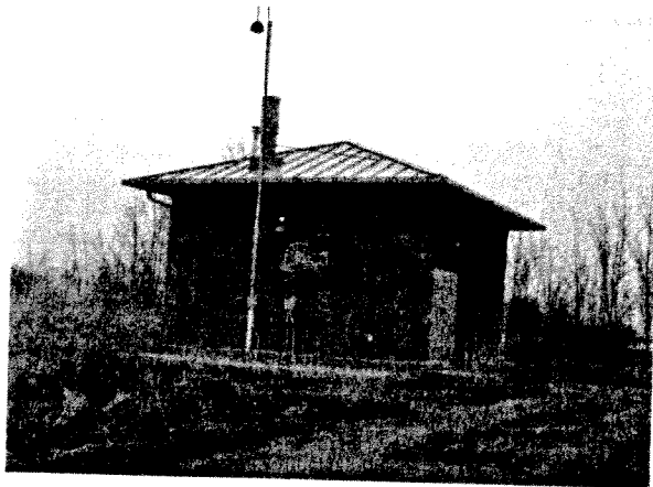
Sanitary Lift Station
