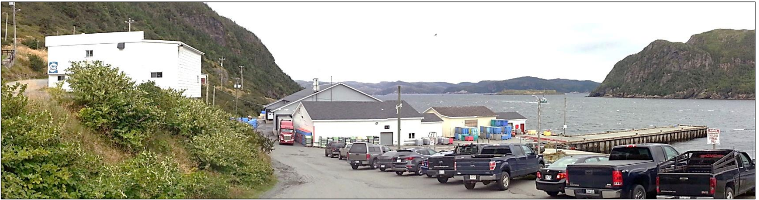
Above: Approach to the subject property along Plant Road. The processing plant is beyond the white federal bait building.
