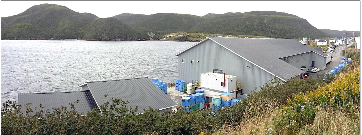
Below: The water treatment facility (left) and processing plant (right) viewed from higher ground on Pointe Road.
