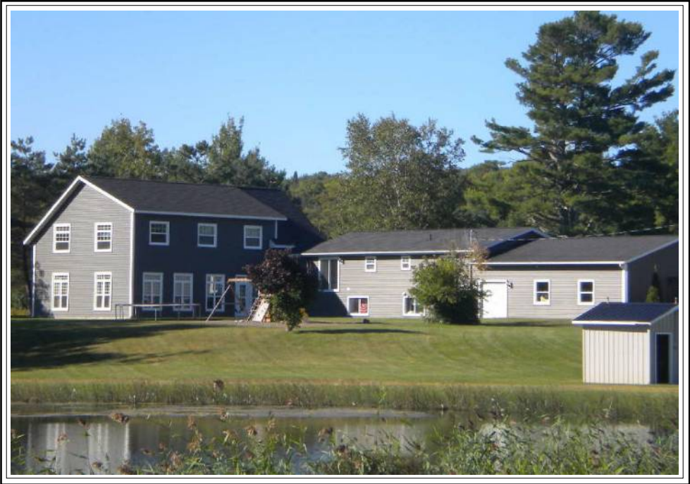
FRONT VIEW OF SUBJECT PROPERTY
