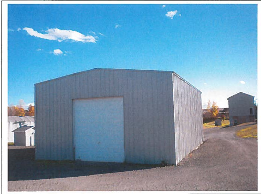
Feed Building ( building 5)
