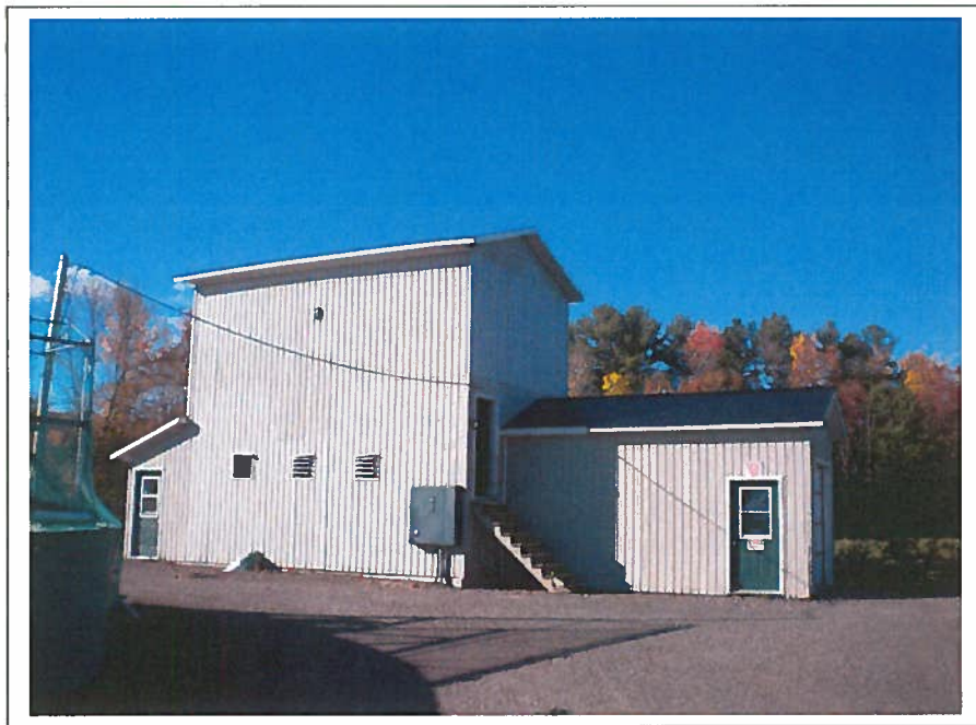
Head House / Chemical ( building 3)
