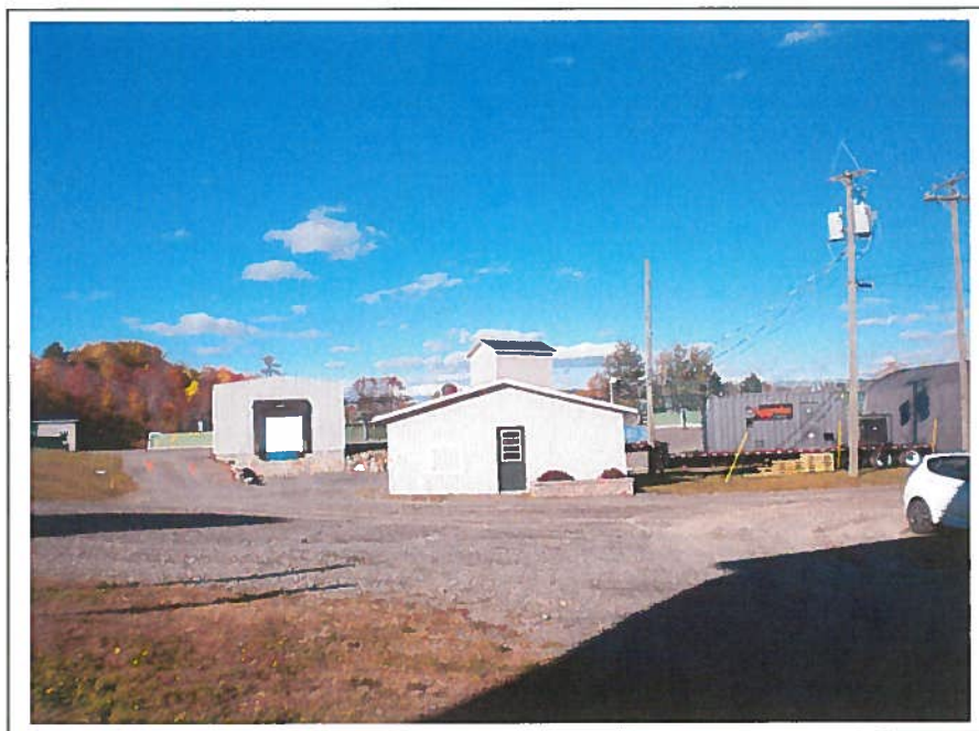
Control Building (building 6)
