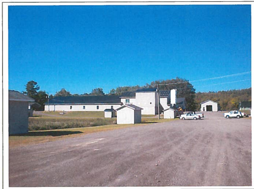
Hatchery/Well Houses/Head House (buildings 1 and 7)
