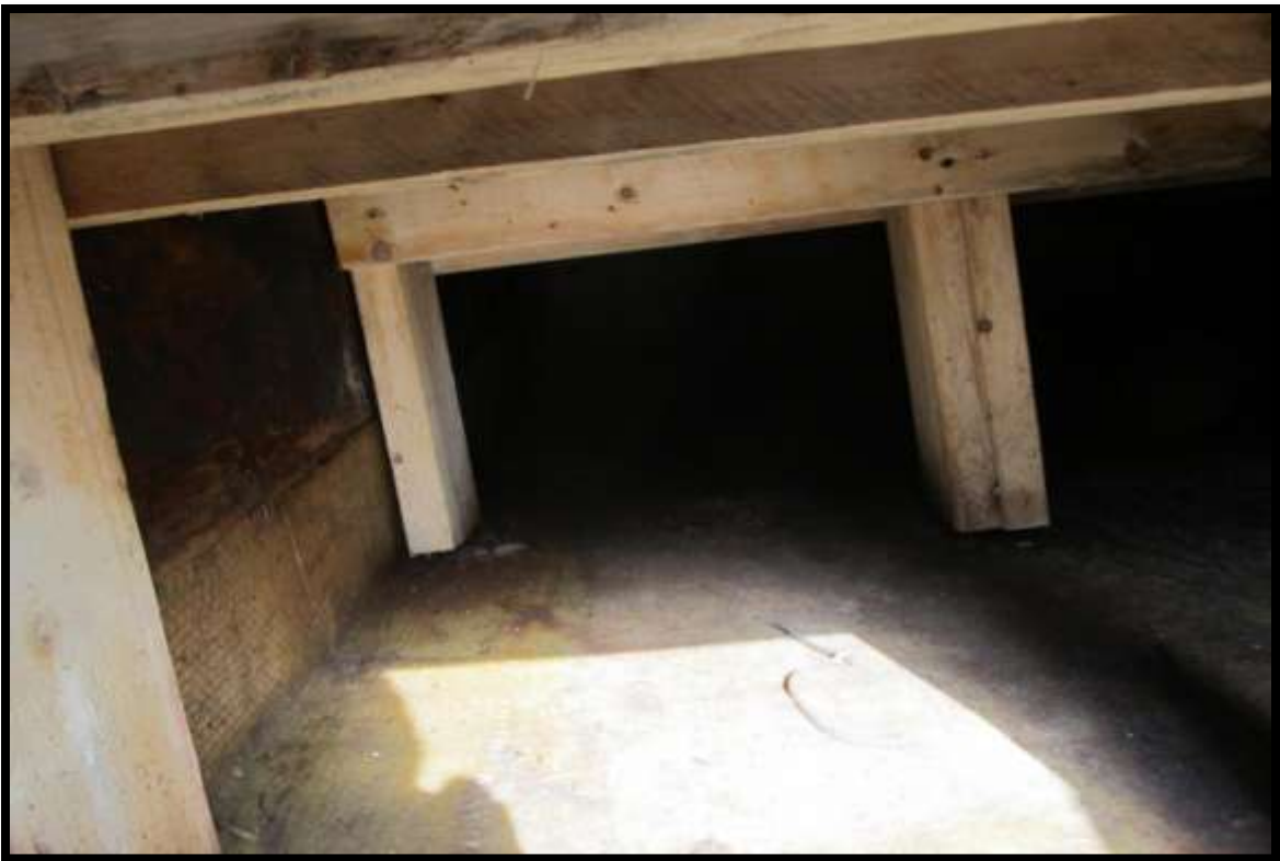
MAIN DECK STRUCTURE
