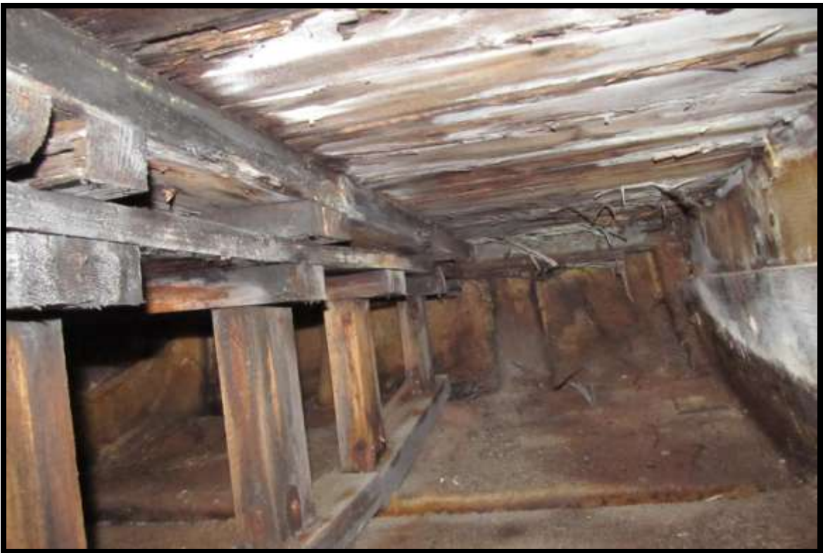
MAIN DECK STRUCTURE
