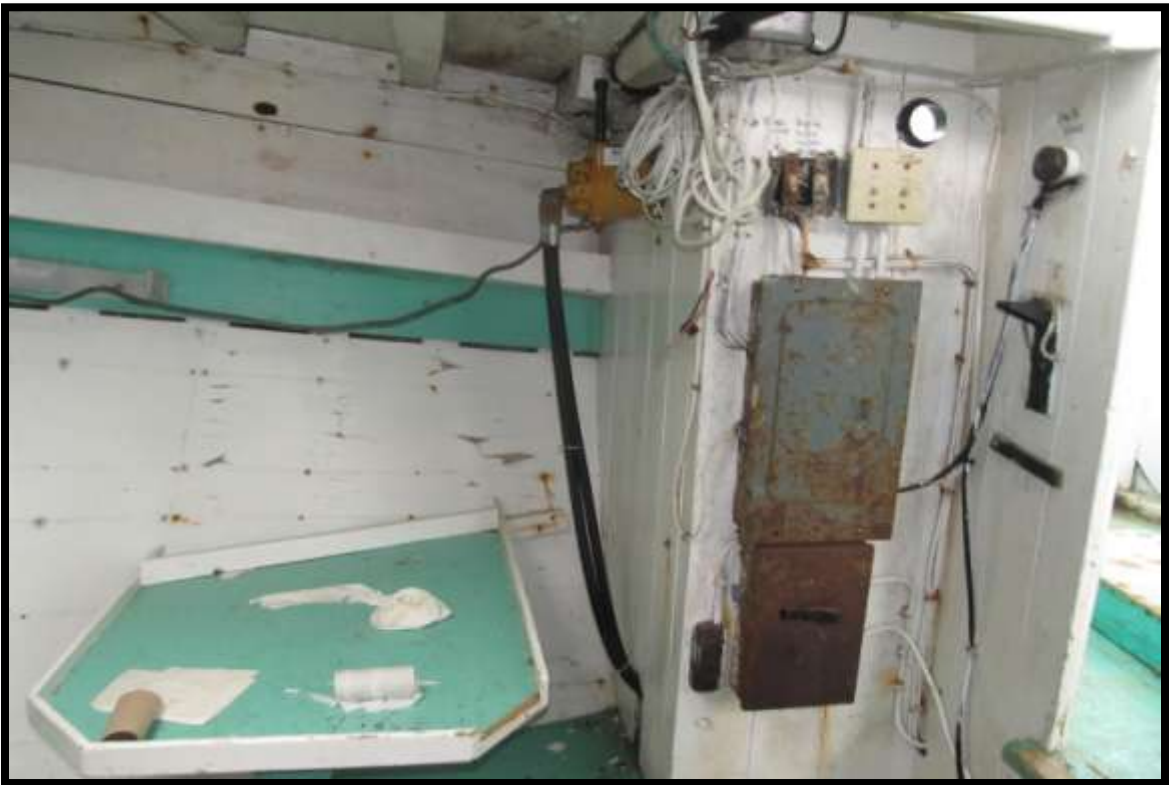
FOC'SLE ACCOMMODATIONS LOOKING STARBOARD
