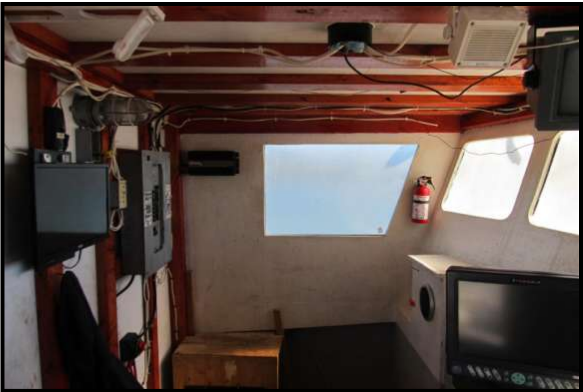
WHEELHOUSE LOOKING PORT
