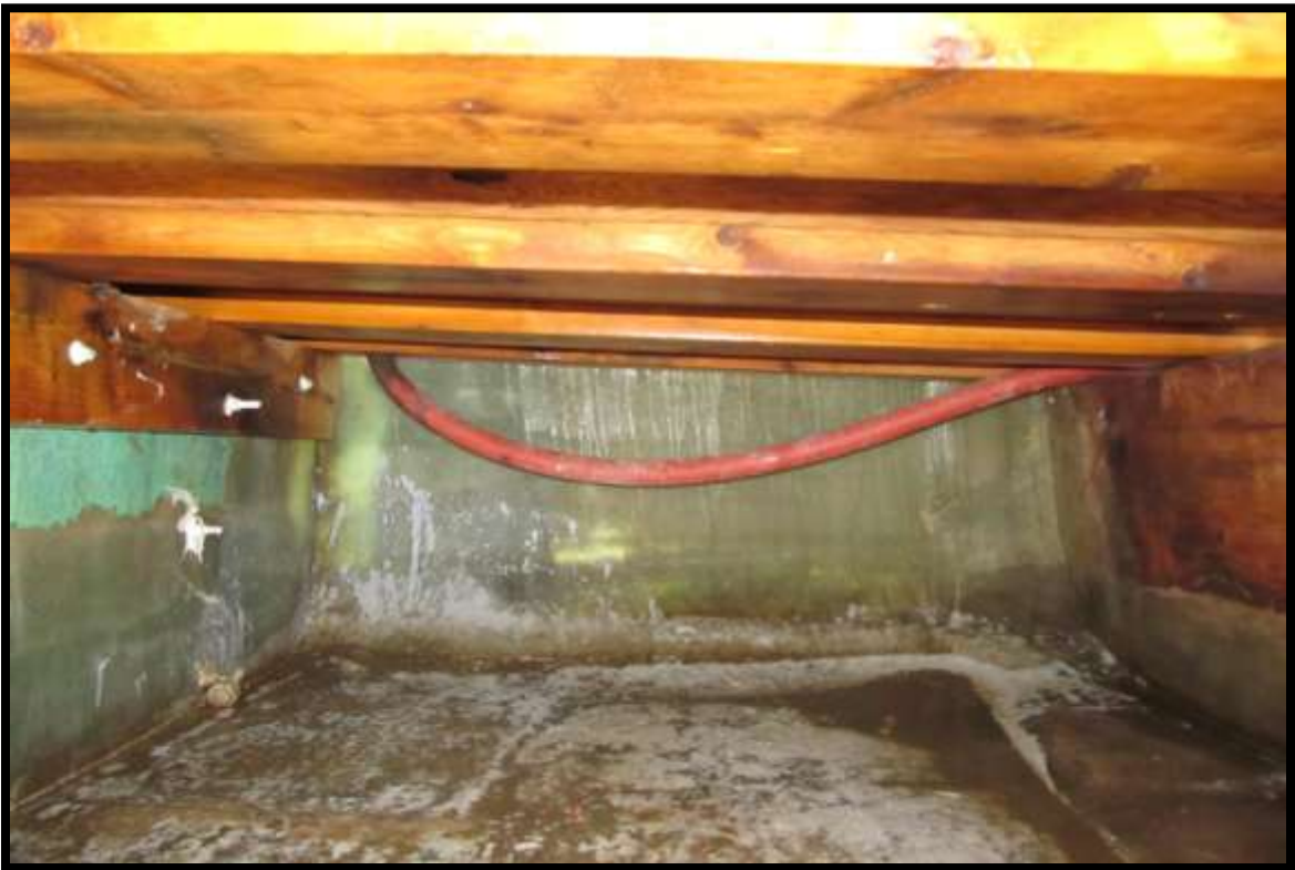
MAIN DECK STRUCTURE
