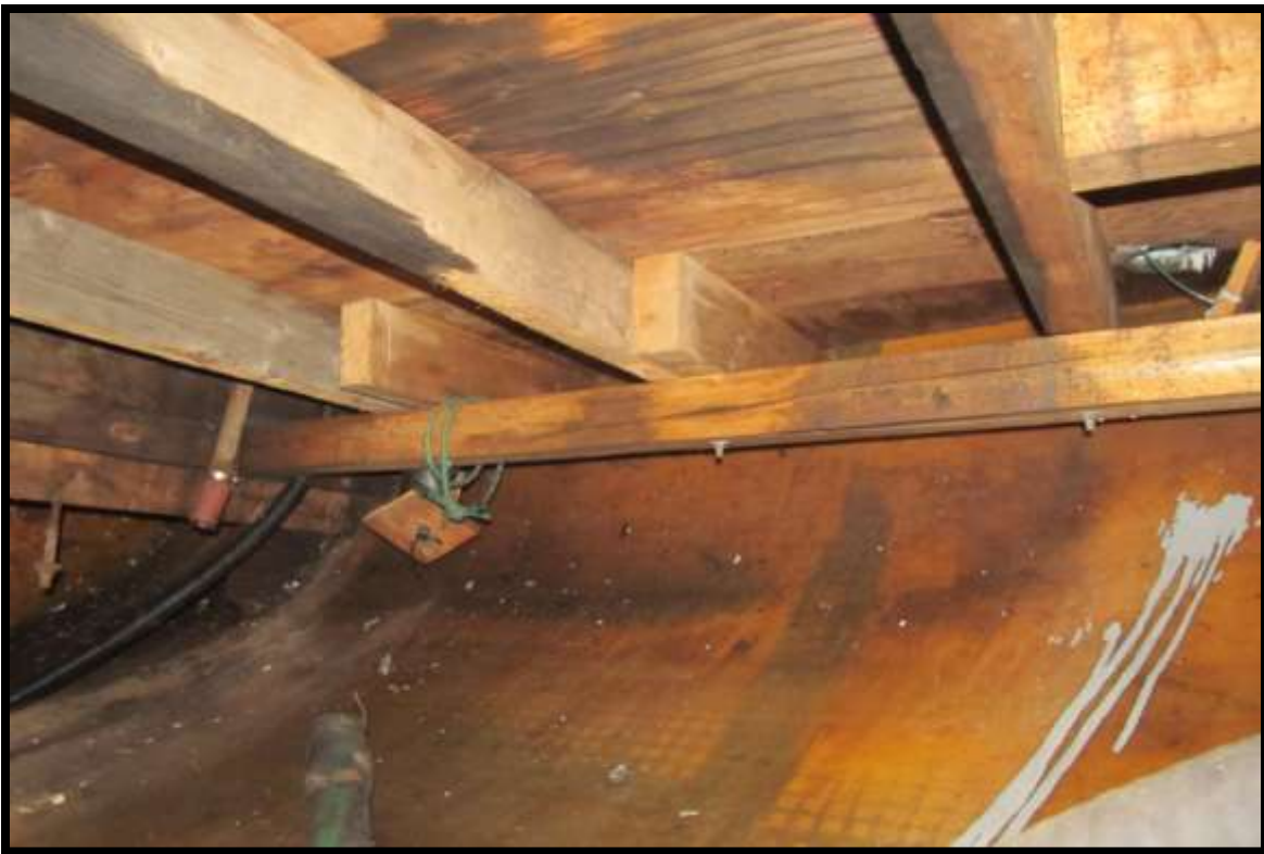
DECK STRUCTURE ON WAY OF ENGINE COMPARTMENT
