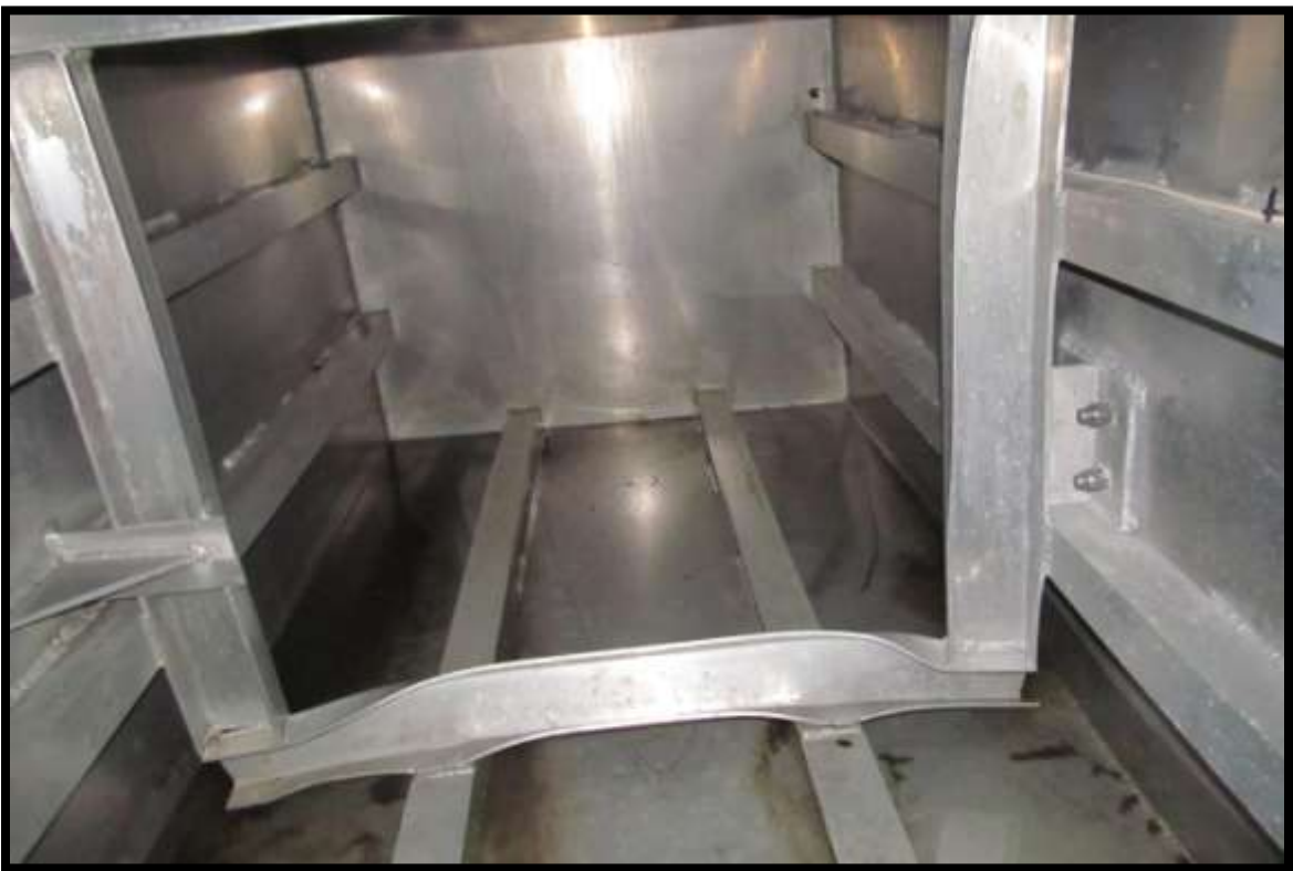
BARGE PONTOON STRUCTURE
