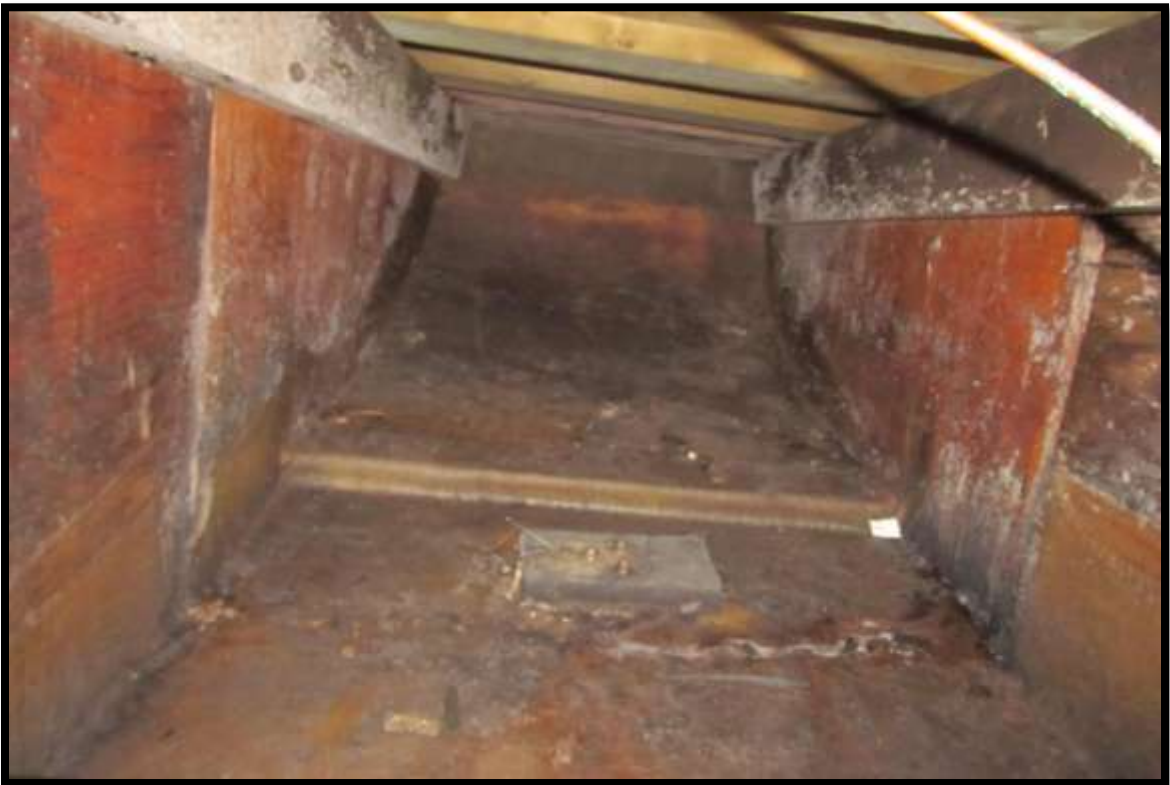
UNDER DECK STRUCTURE
