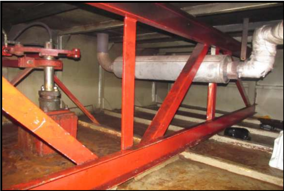
STEERING GEAR AND AFT BARGE STRUCTURE
