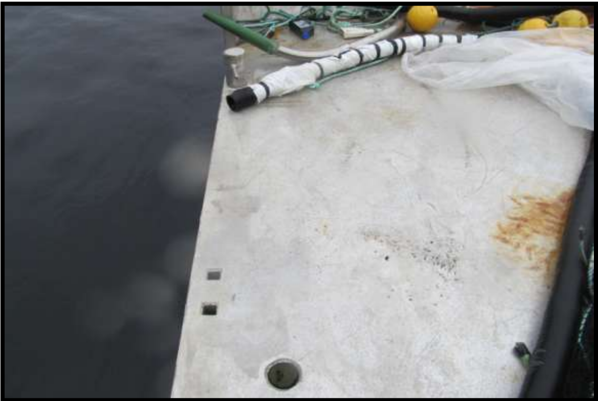
DECK PLUGS AND RAILING POCKETS
