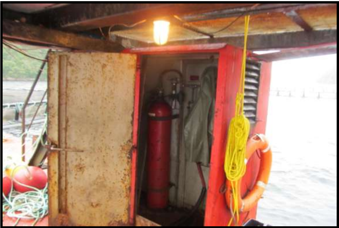
ENGINE ROOM ACCESS
