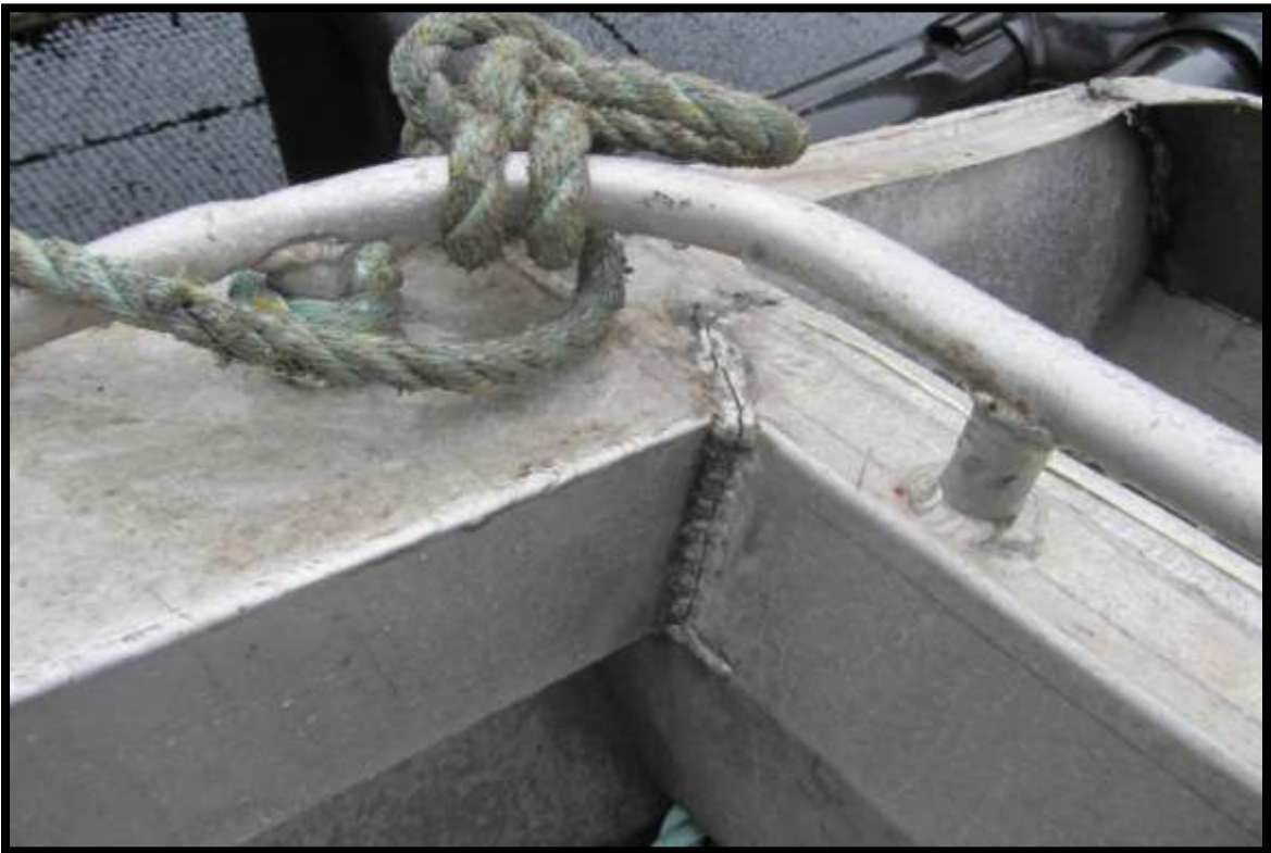
BULWARK WELD FRACTURES
