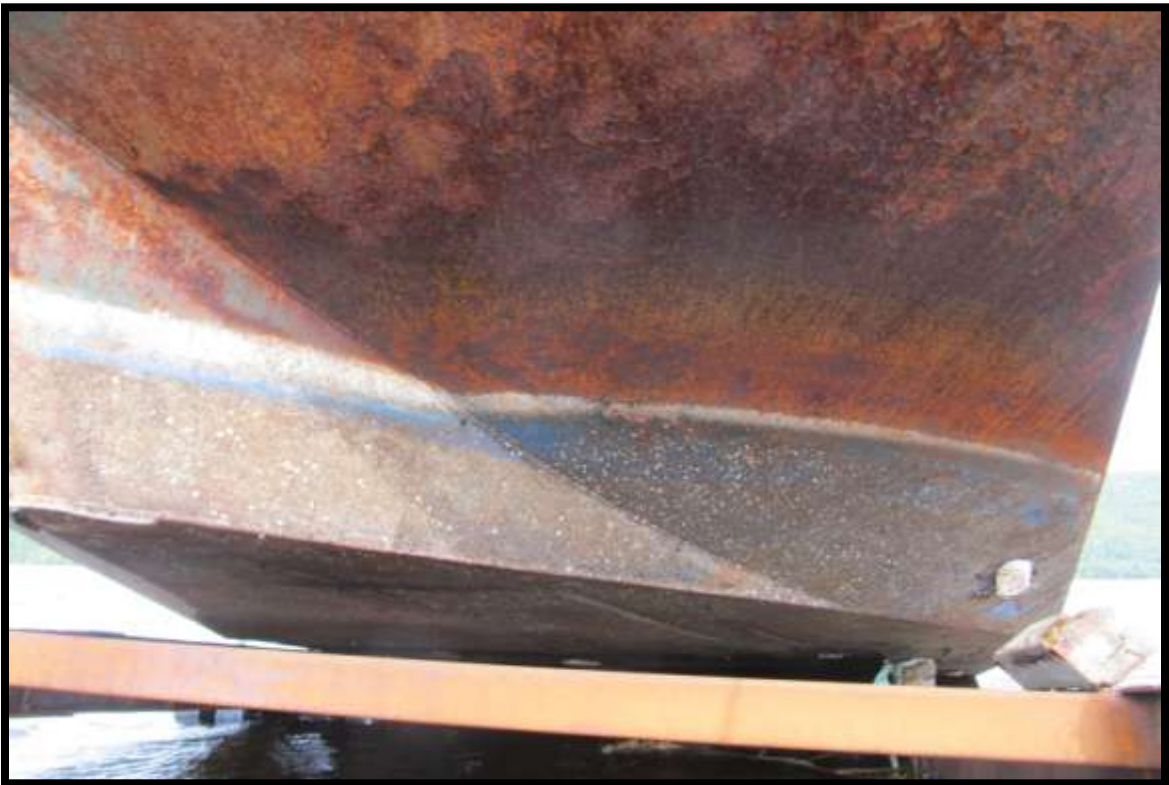
PORT SIDE UNDERWATER HULL (LOOKING AFT)
