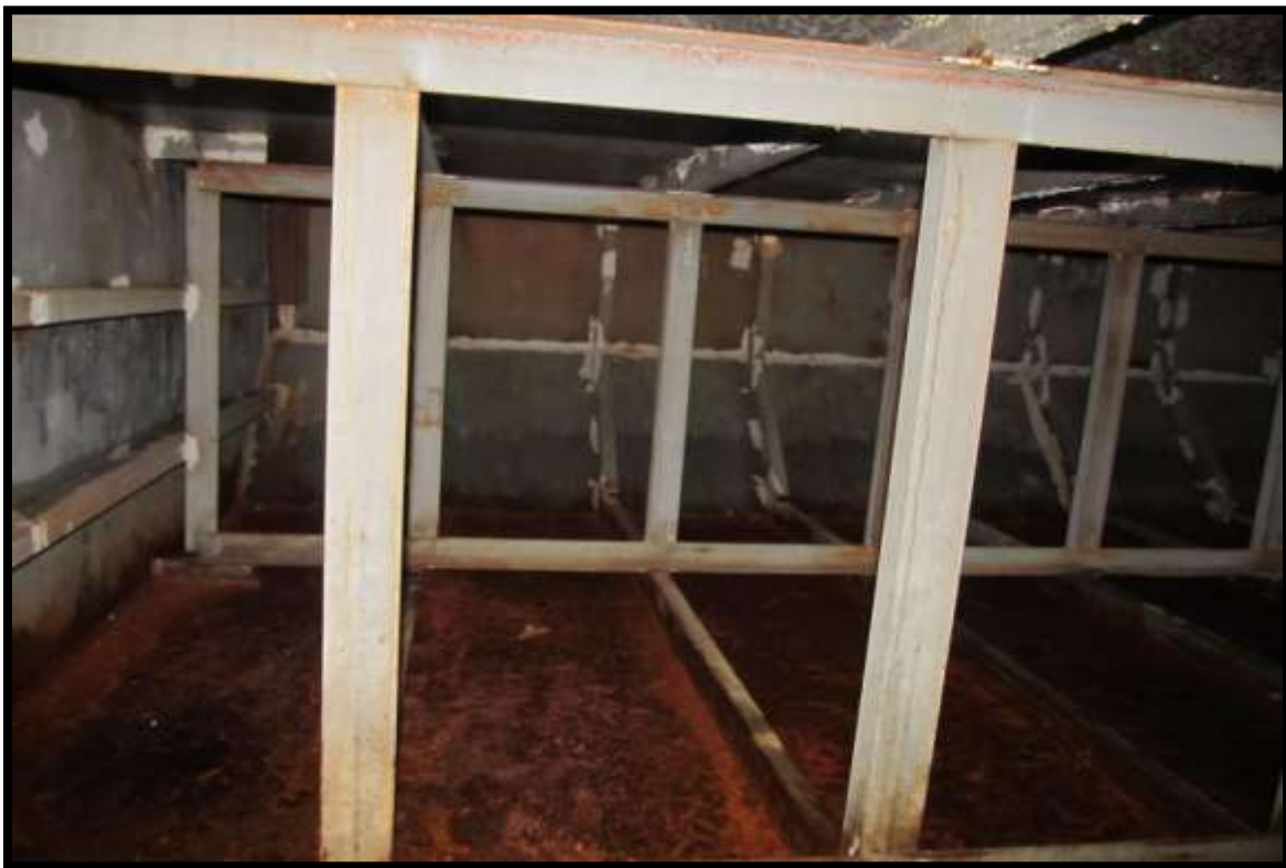
FORWARD COMPARTMENT UNDER DECK STRUCTURE
