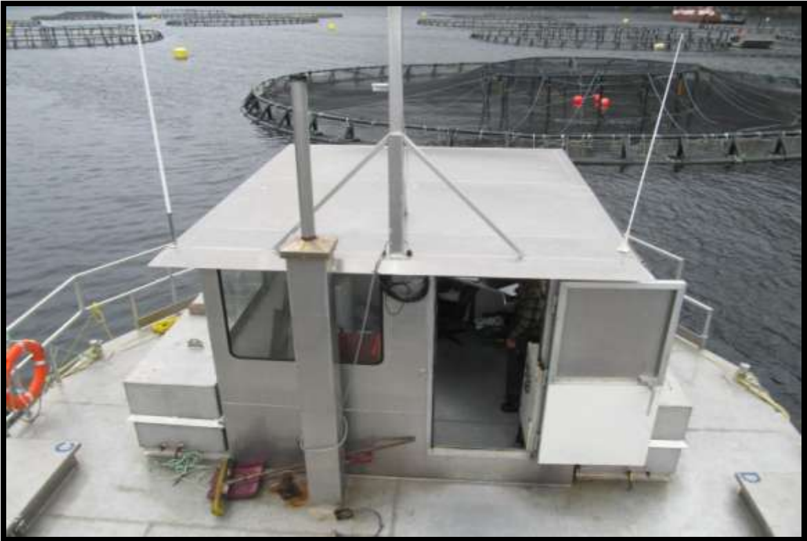
MAIN DECK LOOKING FORWARD – FEED CONTROL STATION
