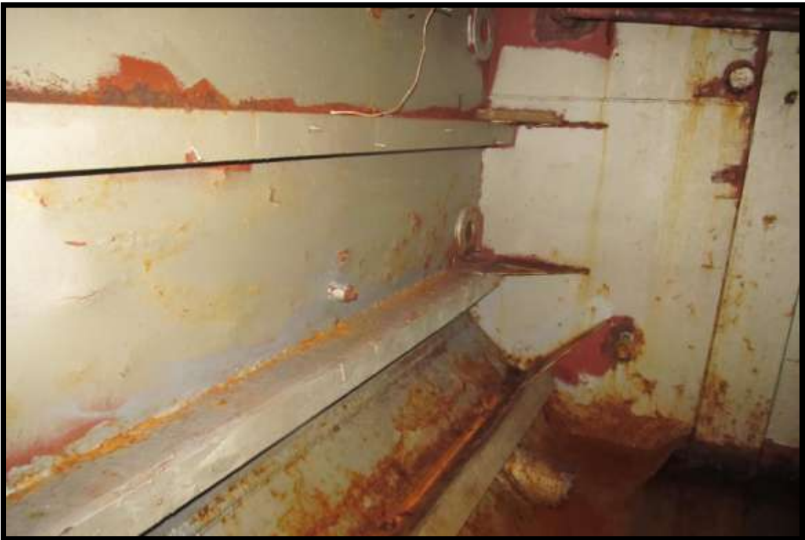
PORT SIDE HULL STRUCTURE
