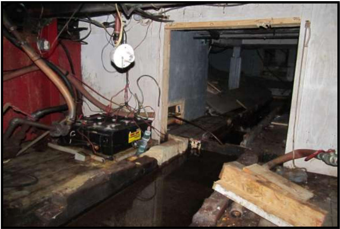
ENGINE ROOM COMPARTMENT LOOKING AFT
