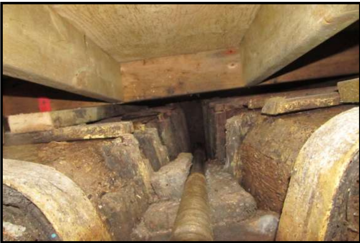
SHAFT TRENCH AND MAIN DECK STRUCTURE
