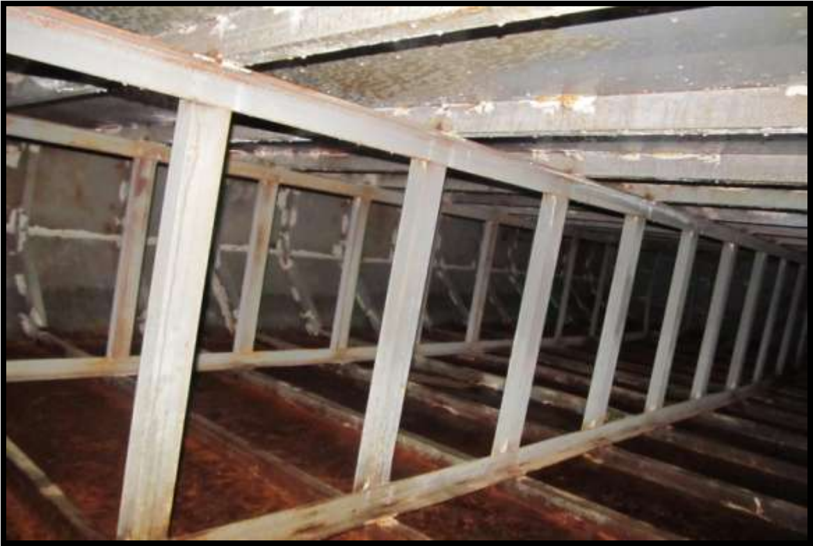
FORWARD COMPARTMENT UNDER DECK STRUCTURE
