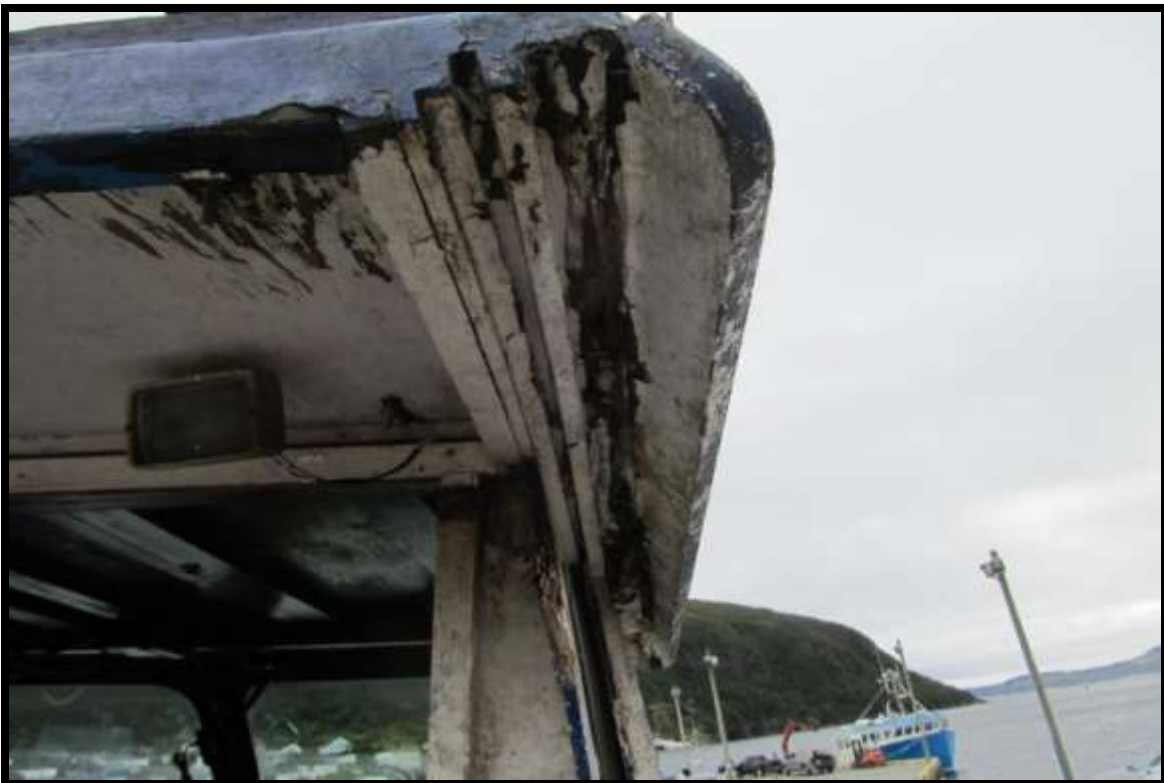
STARBOARD SIDE EAVE AND DECK DAMAGE. EXTENSIVE ROT NOTED
