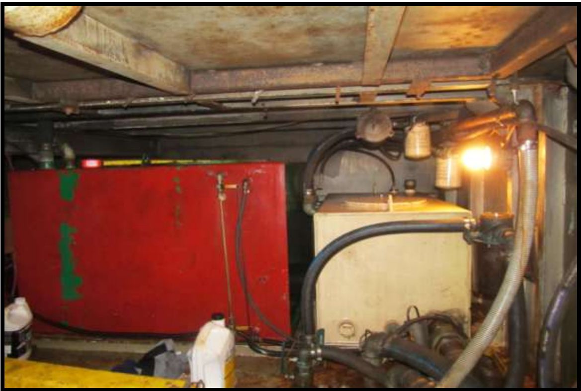
FUEL AND HYDRAULIC OIL TANKS
