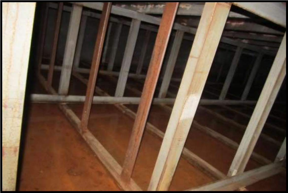
UNDER DECK STRUCTURE
