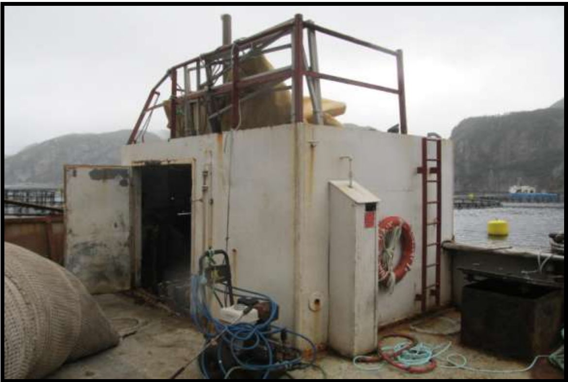
AFT MACHINERY COMPARTMENT
