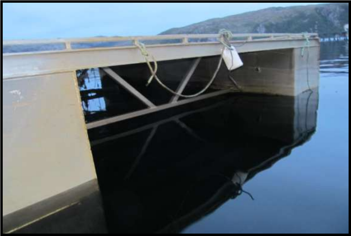
BARGE PONTOONS AND BRIDGE STRUCTURE
