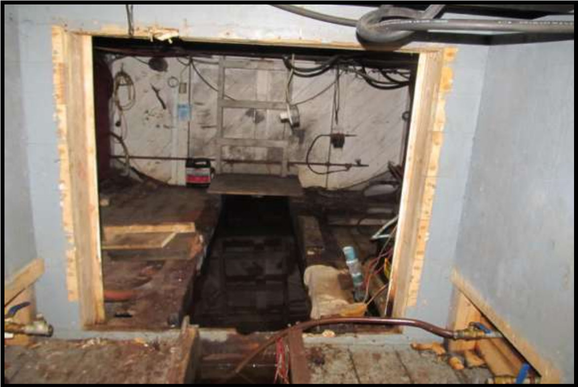
ENGINE ROOM COMPARTMENT LOOKING FORWARD
