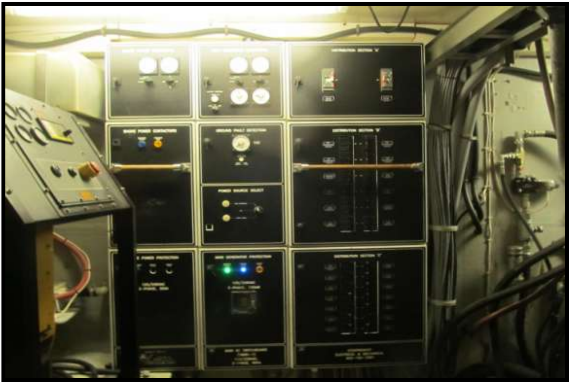
ELECTRICAL SWITCHBOARD
