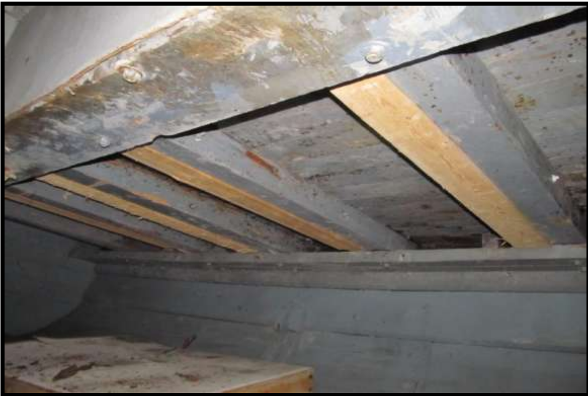
MAIN DECK STRUCTURE WITHIN FISH HOLD.
