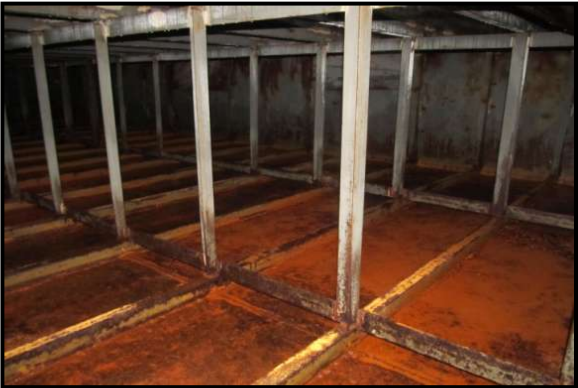
UNDER DECK STRUCTURE
