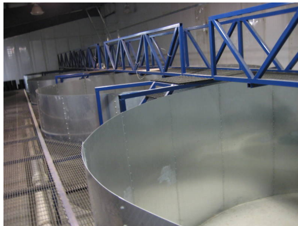
Ref. #20 30-Cu. Meter 20' Dia. x 8'H Bolted Galvanized Steel Panel Broodstock Tanks
