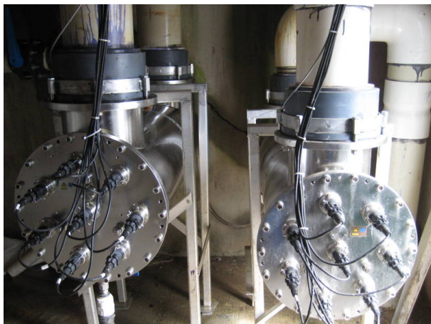
Ref. #25 Wedeco Model BX650, Stainless Steel UV Water Disinfection Systems(New 2004)
