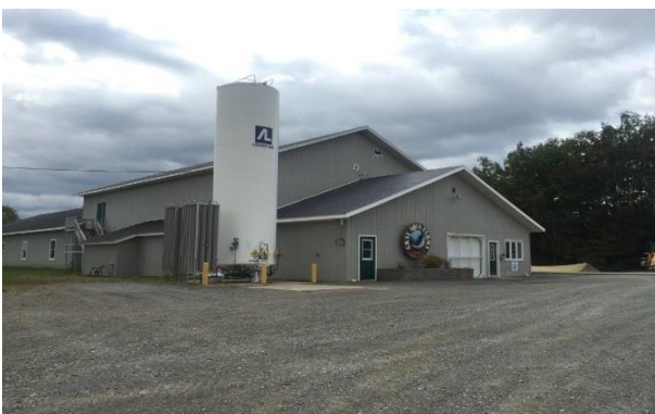
Main View of the Office Building
