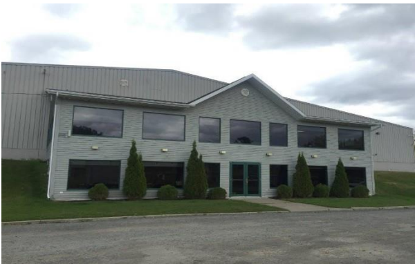
Front View of the Office/Admin Building
