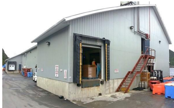
Exterior of the Plant
