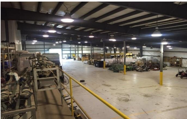
Rear-view from a Mezzaine
