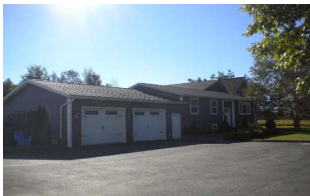
Rear View of the Property
