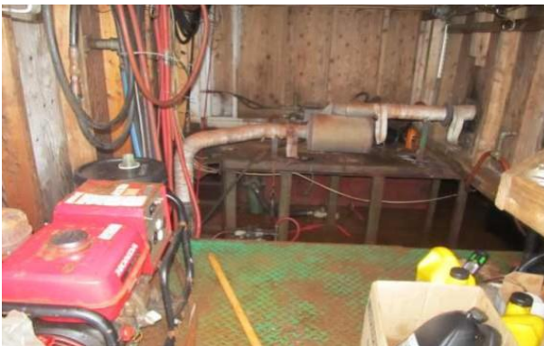
Machinery space below wheelhouse
