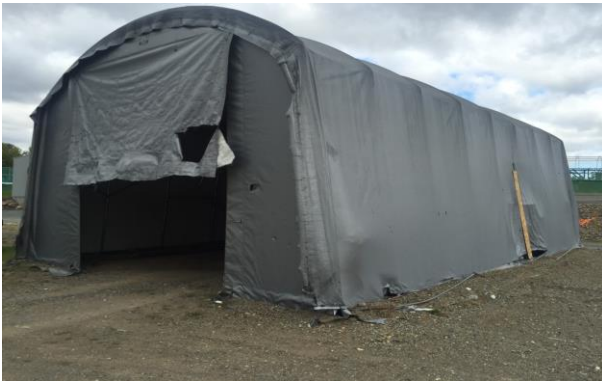
Front View of the Quonset Hut
