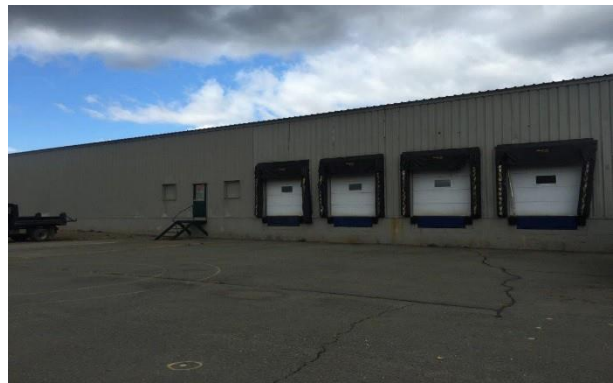
Bay Doors on the Side of the Warehouse
