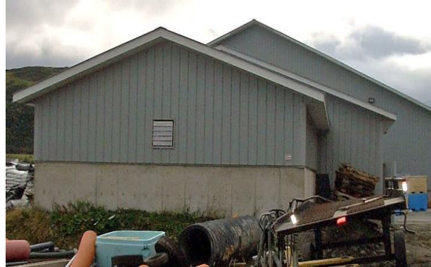
Water Treatment Building (Rear)
