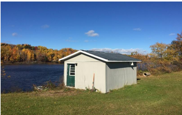
Front View of the River Intake Pump House
