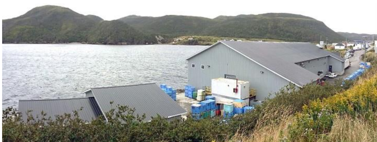
Processing and Water Treatment Plants
