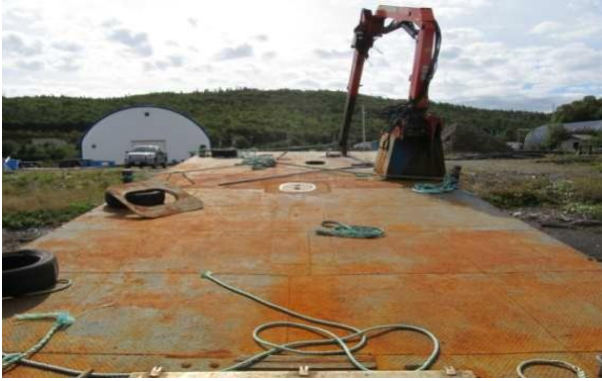
Main Deck Looking Forward
