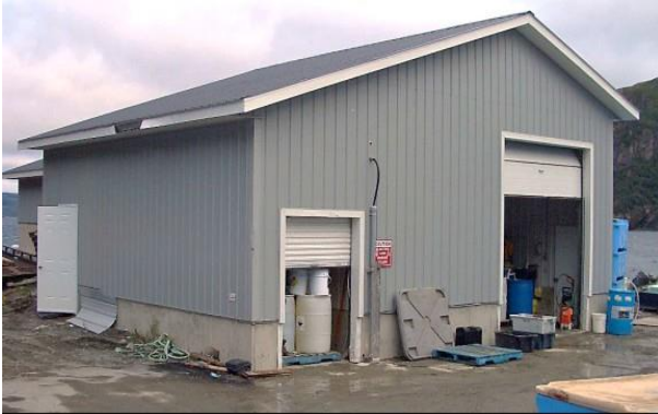
Water Treatment Building (Front)
