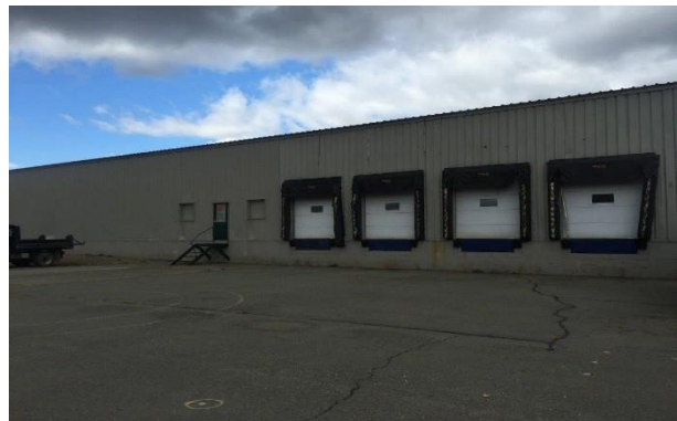
Bay Doors on the Side of the Warehouse
