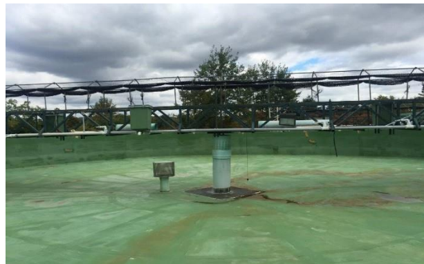
Internal view of a holding tank
