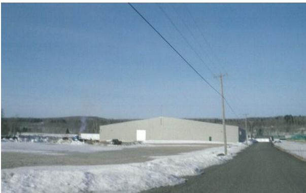
Back view of the Warehouse
