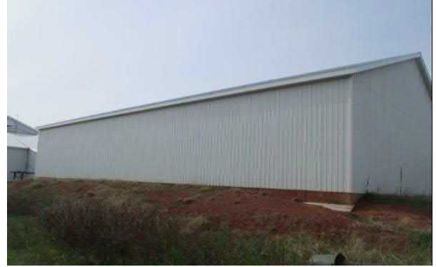
Freezer Building Exterior
