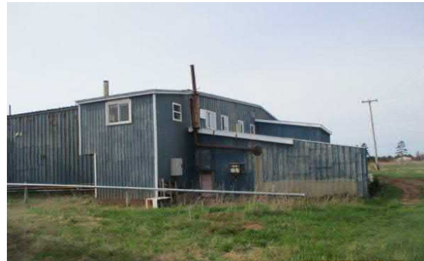
Processing Plant (Side view)
