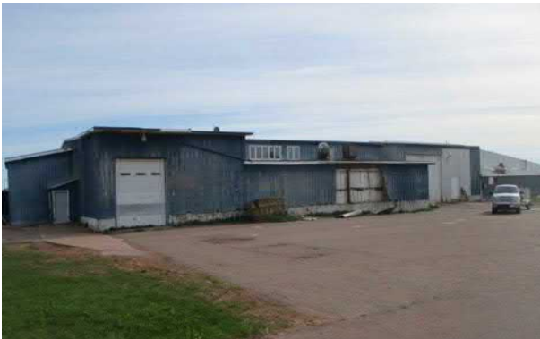
Processing Plant (Front)
