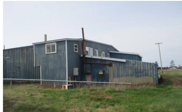
Processing Plant (Side view)
