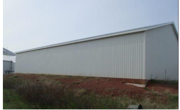
Freezer Building Exterior
