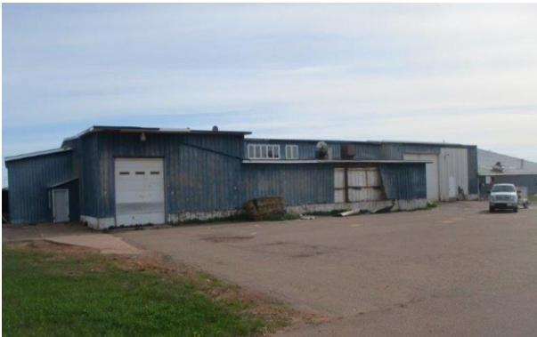
Processing Plant (Front)
