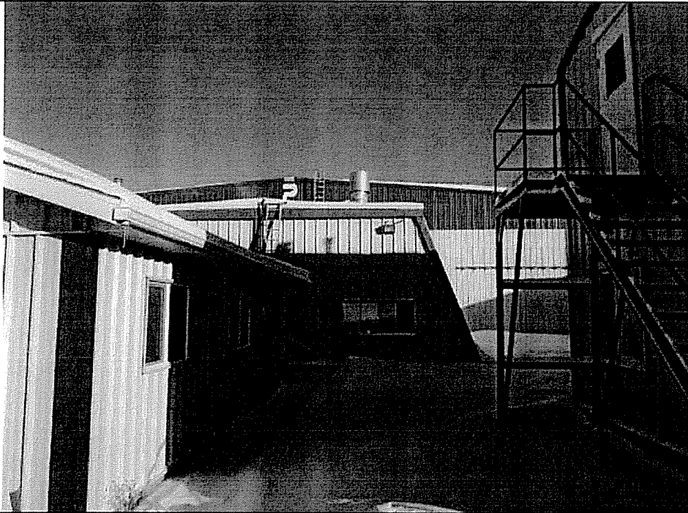
View of Butler Shop/Office Addition
