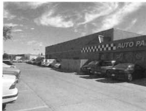
View along West Elevation
