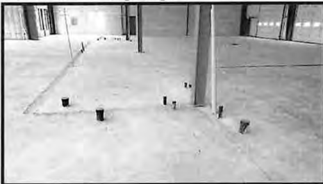
View of the Plumbing Rough Ins
