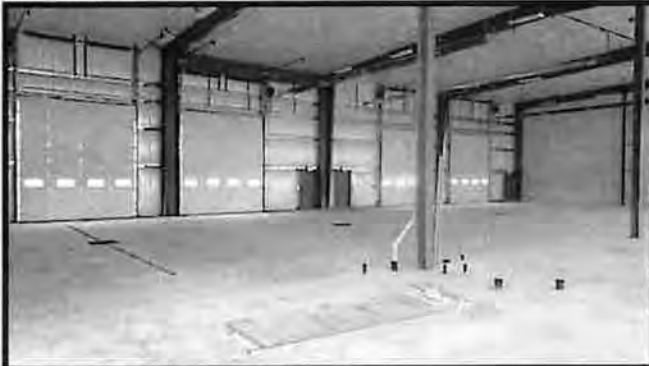
View of the Plumbing Rough Ins
