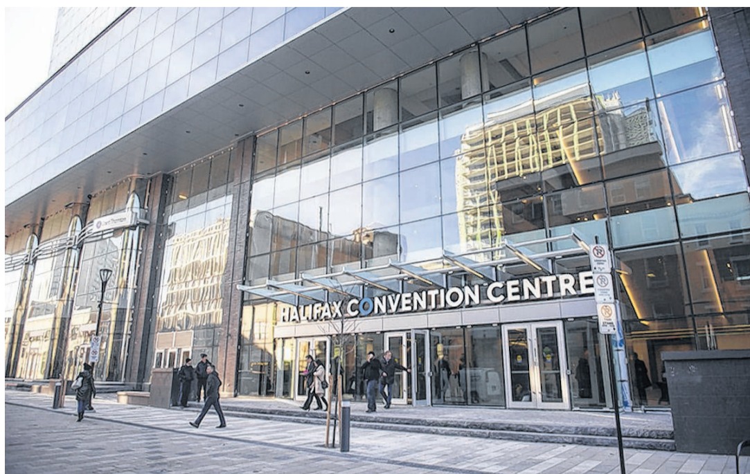
The front of the new Halifax Convention Centre is seen in this December 2017 file photo.
