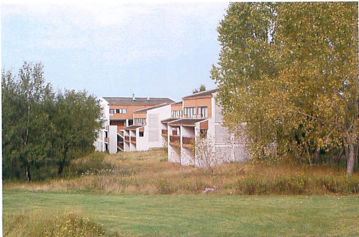
CLUSTER MOTEL UNITS - SPRUCE COURT SOUTH ELEVATION
