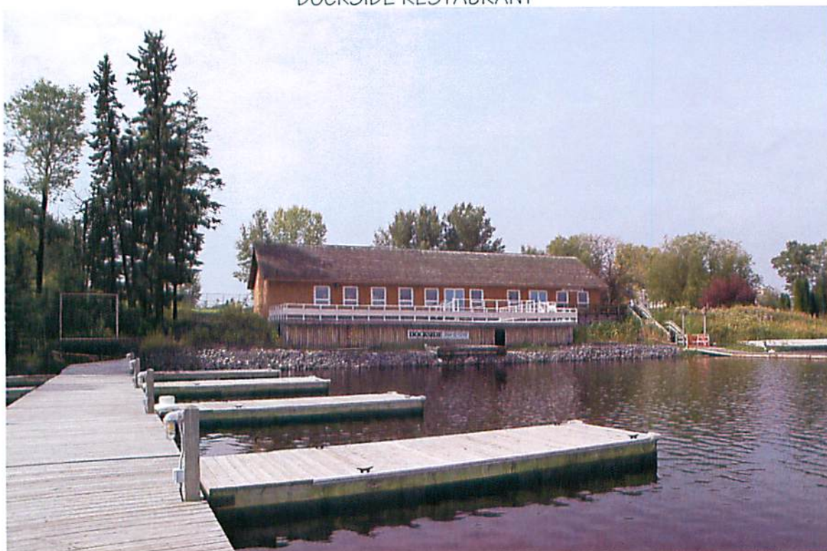
DOCKSIDE RESTAURANT FROM FLOATING DOCK SLIPS
