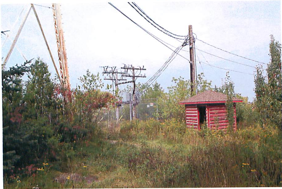
WATER TOWER LEG - TRANSFORMER STATION
