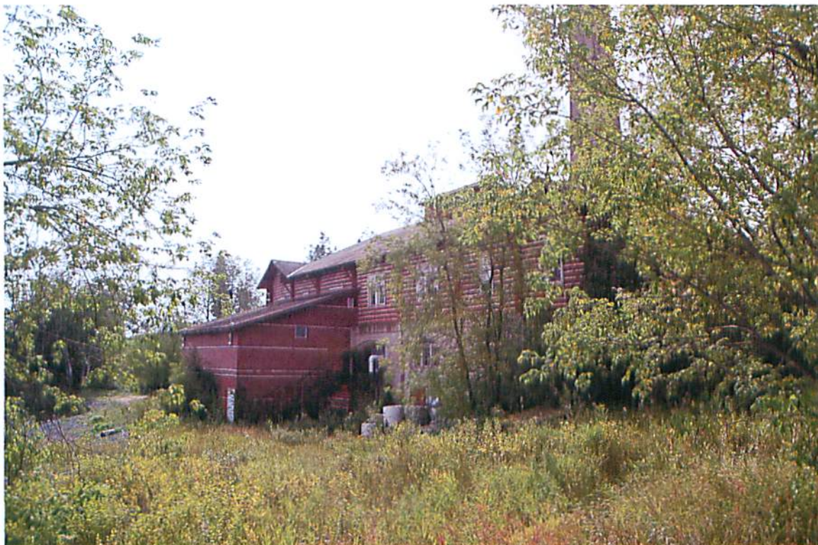
POWER HOUSE - SEWAGE TREATMENT PLANT LOWER LEVEL
