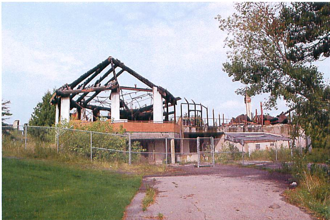
FORMER MAIN LODGE - SOUTH ELEVATION
